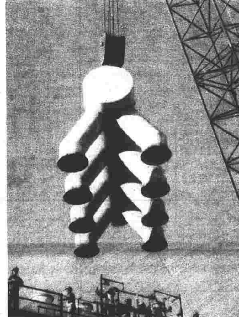
Lower away "Big Bug" is part of a former PPG Industries ethylene glycol production unit shipped from San Juan, P.R., to the firm's Beaumont, Texas, chemical complex, where it will be reassembled. PD Glyco, a joint venture of Pittsburgh-based PPG and the duPont Co. of Wilmington, Del., will operate the relocated plant. PPG and duPont will share the output of the rebuilt unit and an existing plant PPG operates at Beaumont. Total capacity of the combined facilities will be 620 million pounds of ethylene glycol per year. The chemical is used in the production of other chemicals, polyester fibers and in anti-freeze.
